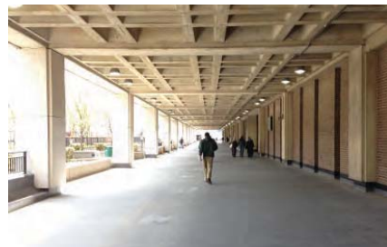
Figure 3.25: Existing Exterior Corridor on First Floor
